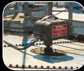
Measuring carbon black in a rubber belt plant.
